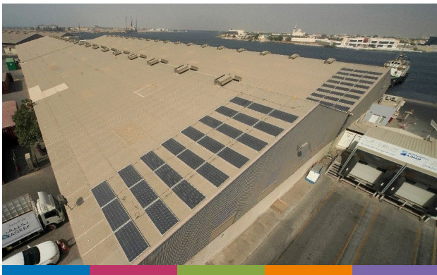
Solar Panels installed on the roof of warehouse in Hutchison Ports Ajman in UAE.
